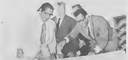
Lt. Governor F. J. Tromp uses trowel to secure cornerstone he laid for 2nd Holiday Inn, witnessed in the center by Holiday Inn's top man Kemmons Wilson.
